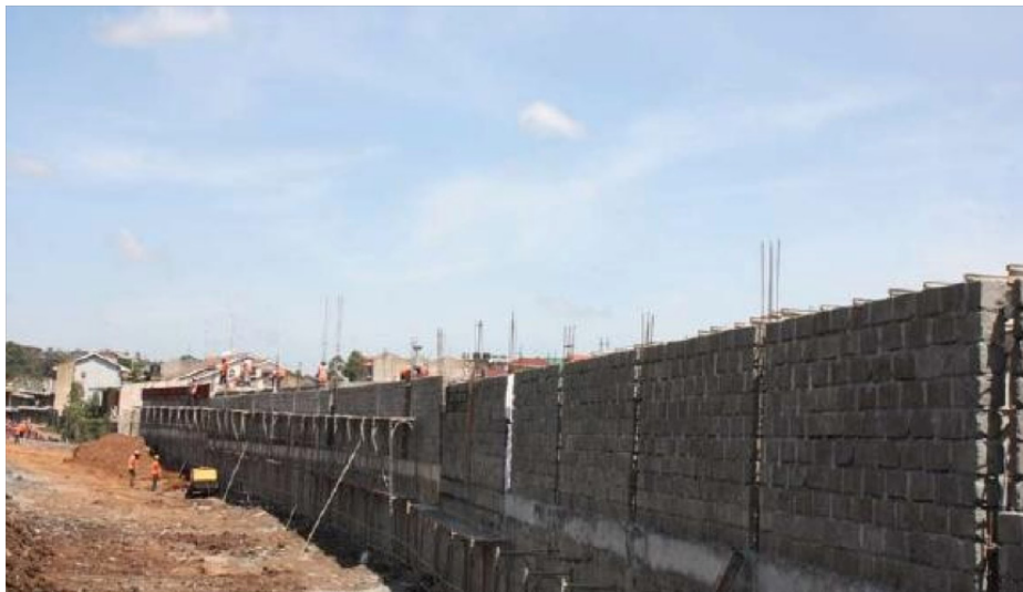
Figure 4: Construction of wall and houses around the Kenya Railway Land in Kibra. Source: Pamoja Trust
